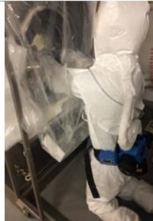
Heal scraping at door opposite discharge
