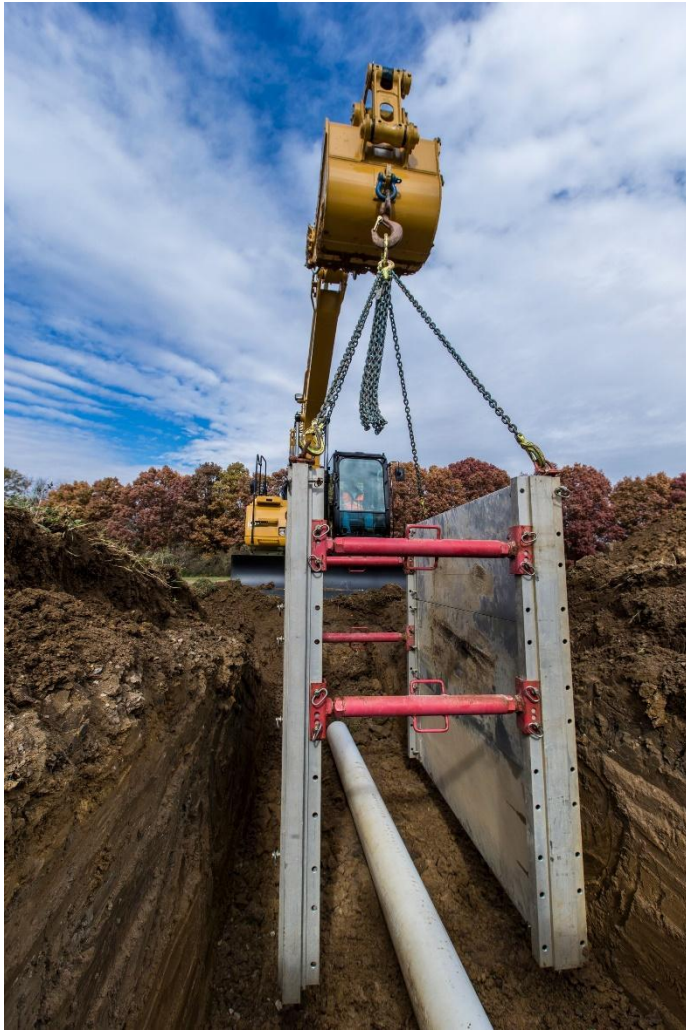
Photo showing a trench box lowered or moved in a trench
