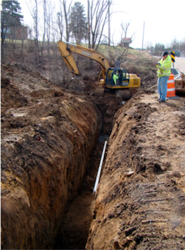
Photos of a deep unprotected trench and a trench with a collapsed wall of soil
