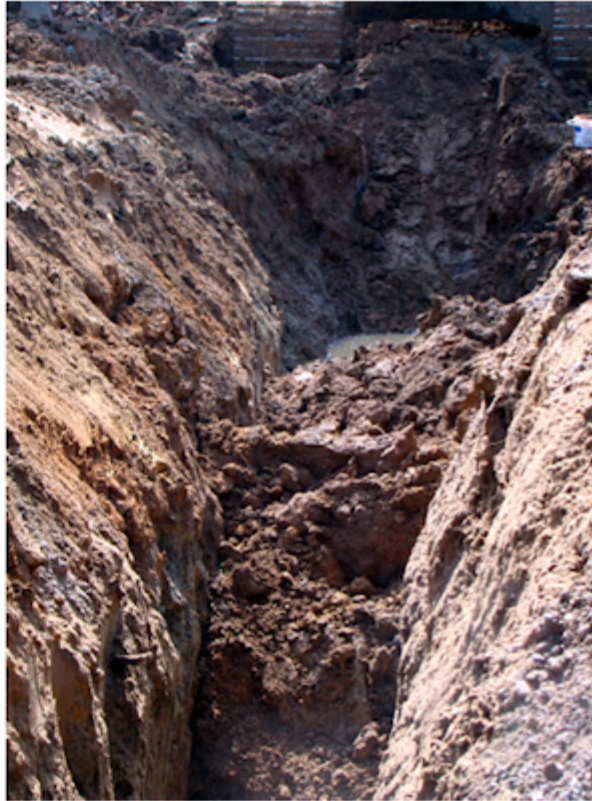
Photos of a deep unprotected trench and a trench with a collapsed wall of soil
